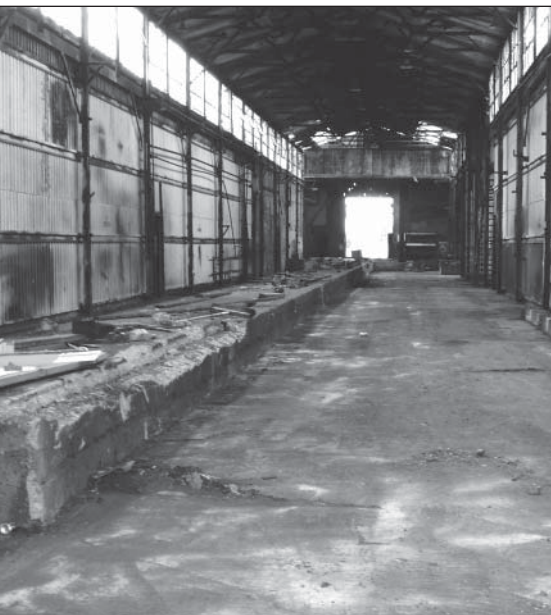
TOP: The paint building on the Derby Tank site in Meade County after the soil cap and new fencing were installed.
